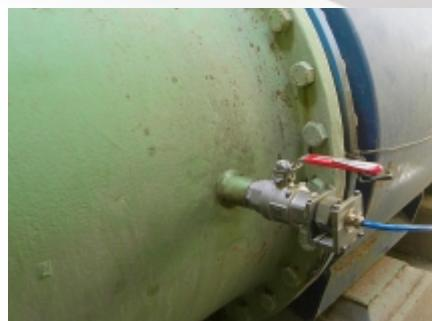
We provide suitable accessories such as welding nozzle, stop ball valve for easy sensor installation and maintenance.
