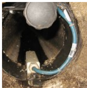
Water-ultrasonic and hydrostatic measurement – for detection of medium discharge ranges e.g. precipitation discharge measurement
